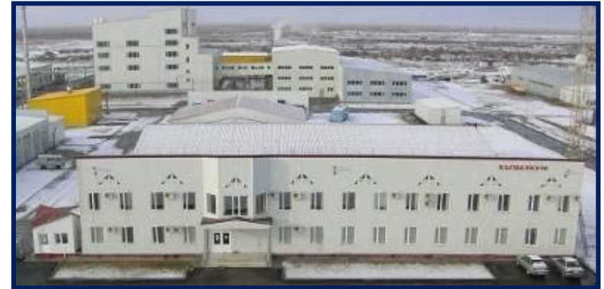
Processing facilities at Kharasan
