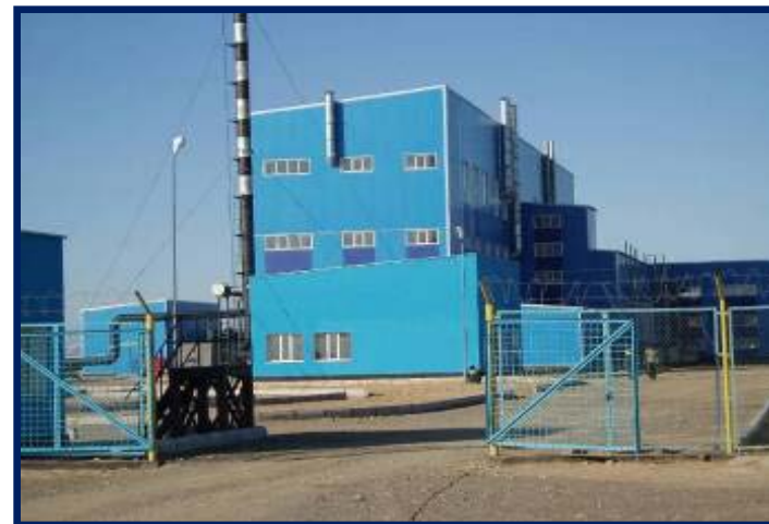
South Inkai production facilities
