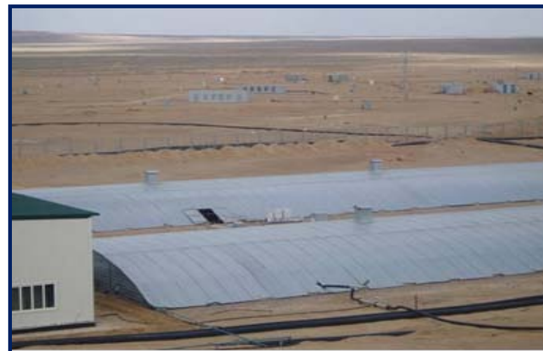
Karatau Well Fields (view from processing plant)
