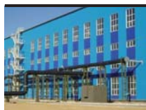
Processing Facility, South Inkai
