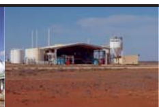
Demonstration Plant, Honeymoon
