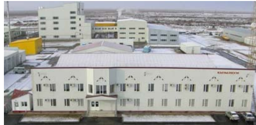
Processing facilities at Kharasan
