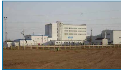
Akdala processing facility
