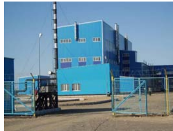
South Inkai production facilities
