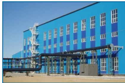
South Inkai production facilities
