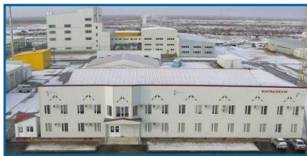
Processing facilities at Kharasan
