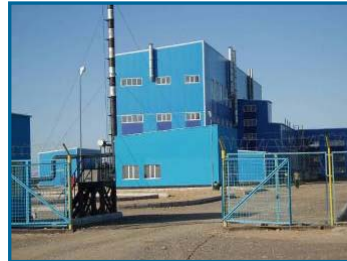
South Inkai production facilities
